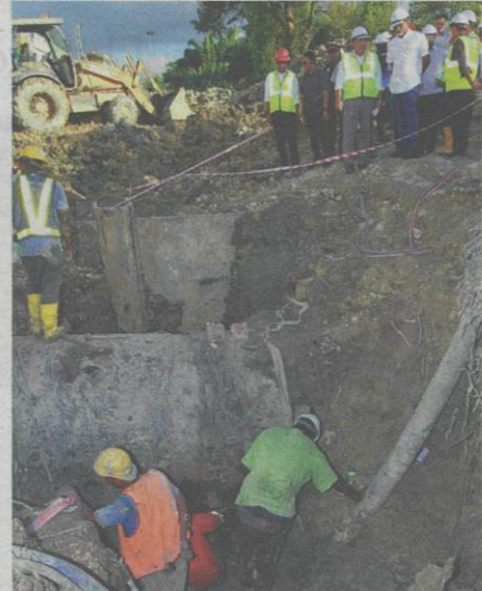
Repair in progress: Dr Xavier visiting the site of the ruptured pipes in Klang.
